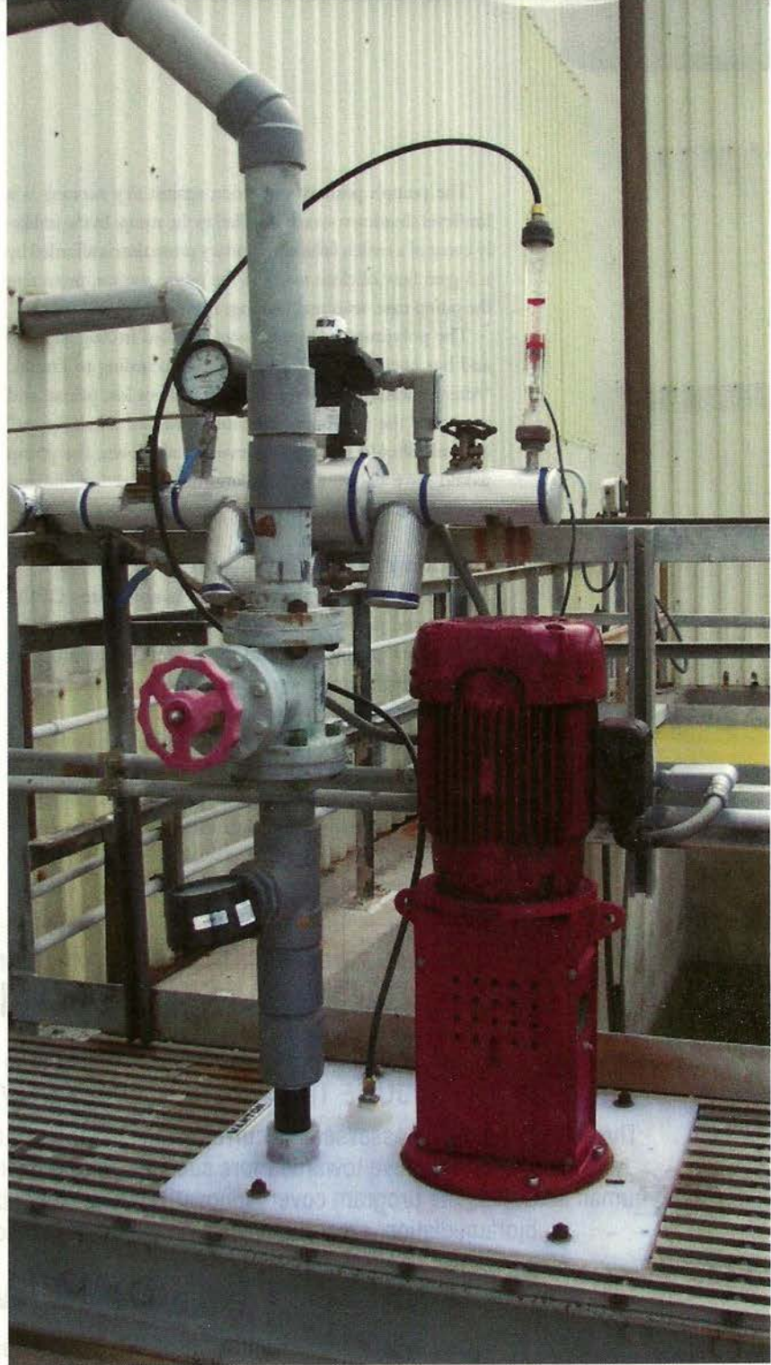
The cantilevered design of Vanton's SGK PY1200 sump pump eliminates wetted bearings, allowing indefinite run-dry capability and reliable starts following extended idle periods. All wetted components are made of solid CPVC, which is abrasion resistant, and inert to the broad range of acidic and caustic fluids collected.
