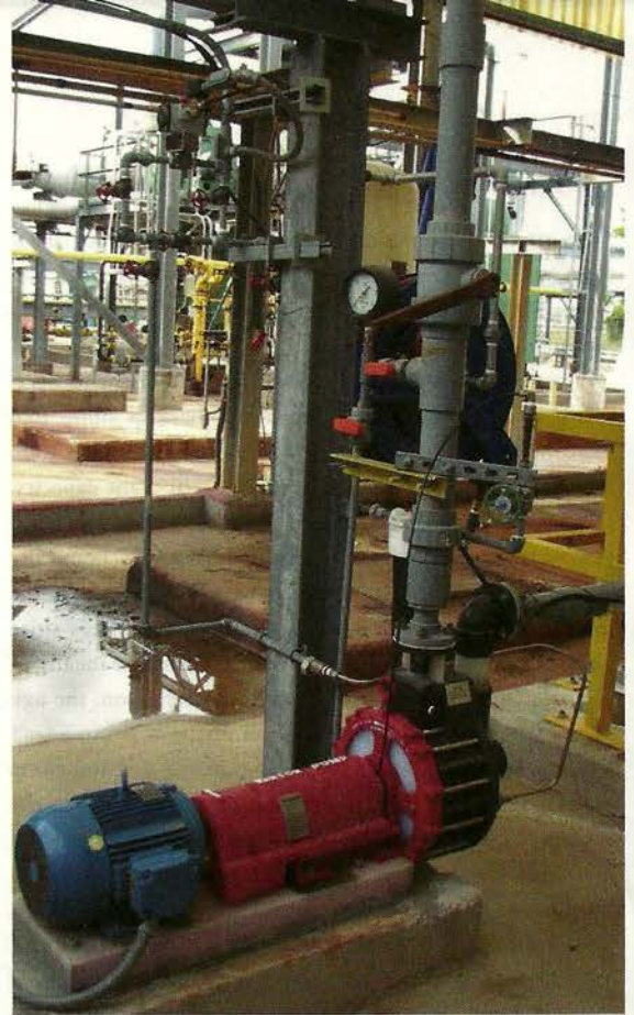
Vanton's Prime-Gard PY450 horizontal self-priming thermoplastic centrifugal pump efficiently transfers demineralizer effluent.
