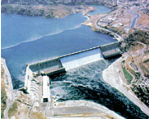
Mechanics of the Grand Coulee Dam incorporated six Vanton sump pumps to ensure reliability and operation of three 805 megawatt turbines.
