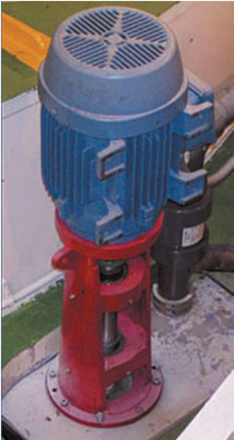
Close-up of one of the six Thermoplastic Cantilever SGK sump pumps with dry-run capability.
